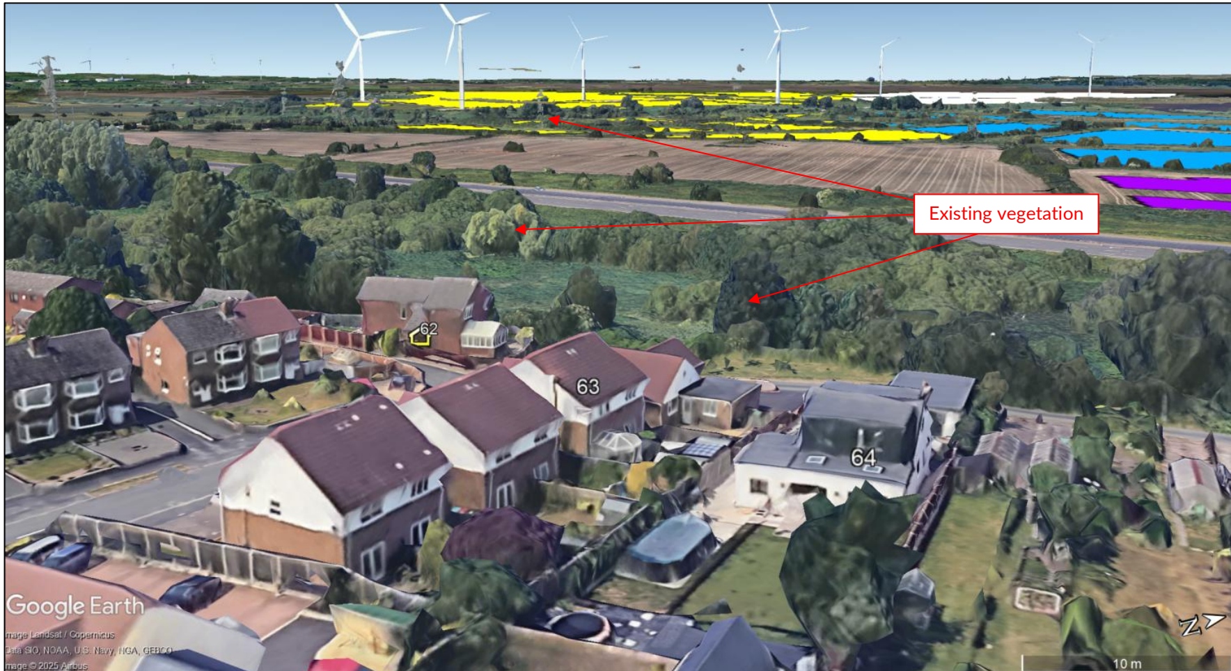
Figure J7775 Reflecting panel area and partial screening for dwelling receptor 62 to 64
